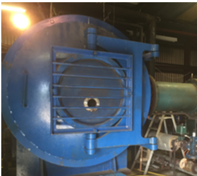
Figure 10: Nammo's F1 thruster facility.
